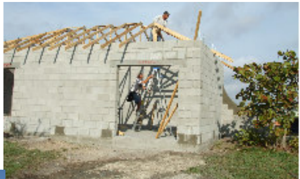
the rafters are put in place...
