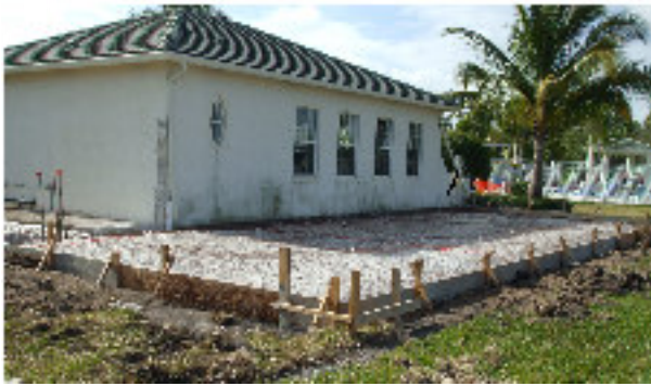
Base for the picnic area is set
