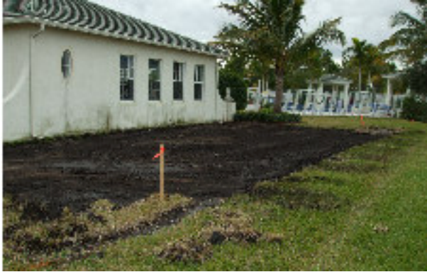
Ground for the picnic area is cleared
