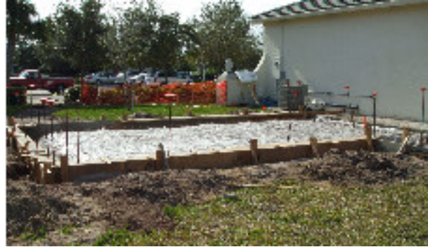
Base for the storage building is set
