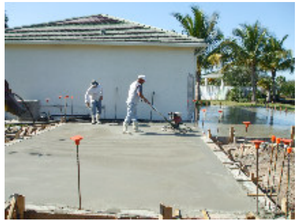
A worker smooths the pads after the concrete has been poured
